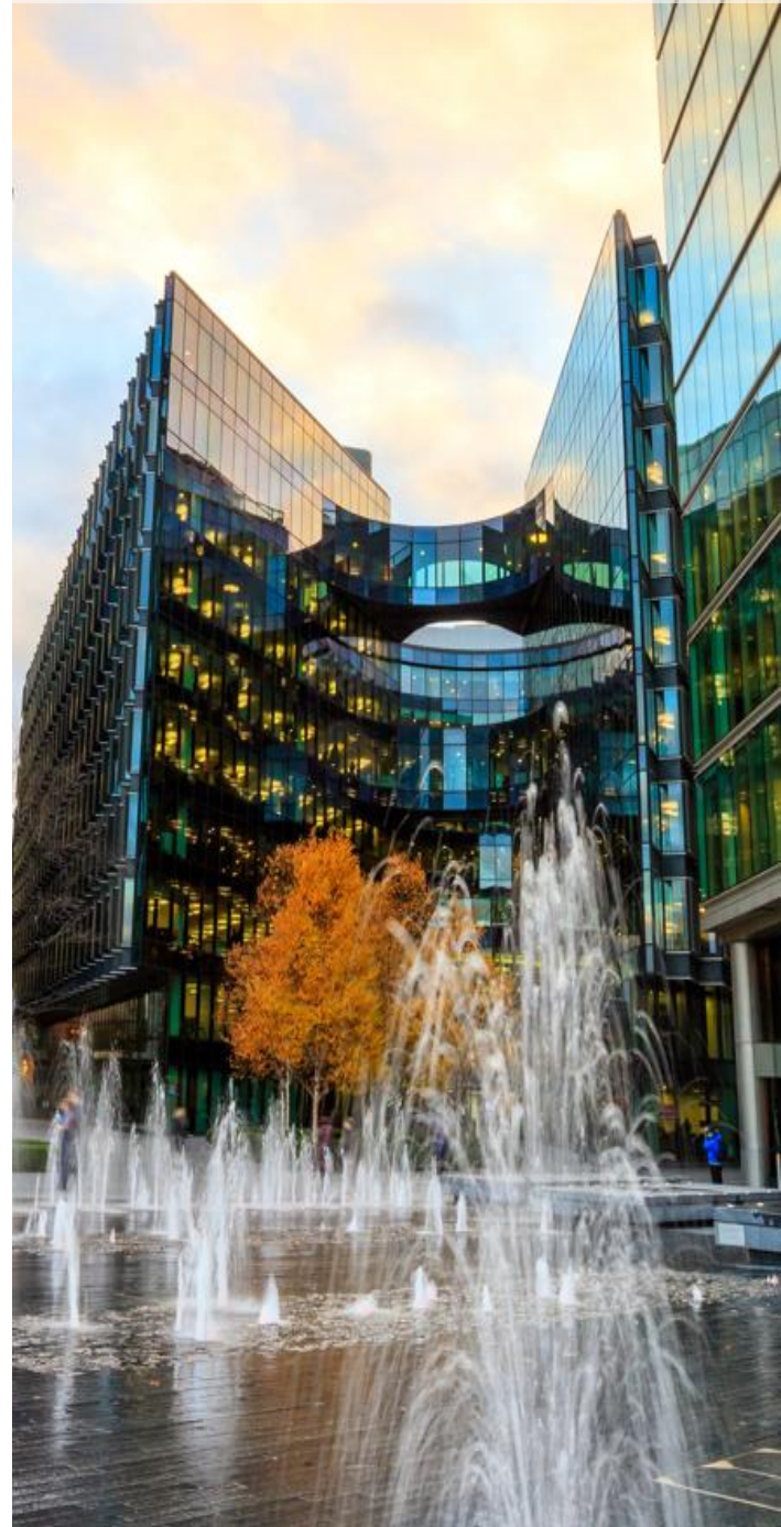
7 More London Riverside - the first office building in England to achieve BREEAM 'Outstanding' accreditation
